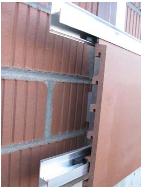
The ArGeLite<sup>®</sup>-H-System substructure consists of horizontal aluminium carrier rails. EPDM-distance pieces keep the tiles in position and guarantee a 4mm vertical joint.
