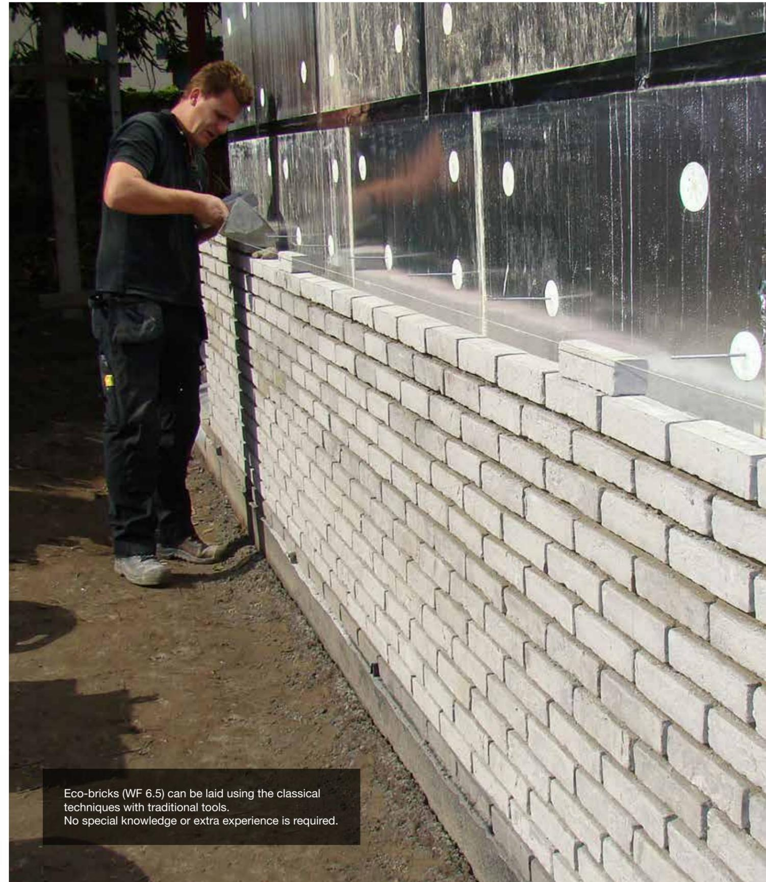
Eco-bricks (WF 6.5) can be laid using the classical techniques with traditional tools. No special knowledge or extra experience is required.
