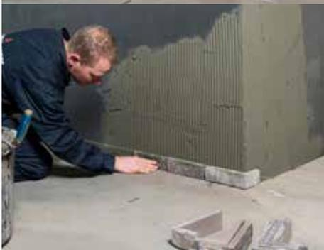
Press the slips into the mortar using a sliding motion. Make sure that the area is almost 100% covered to avoid frost damage. On substrates where the adhesion is poor, or if required for the specific type of mortar, applying a layer of the adhesive to the brick slips themselves can be advisable.
