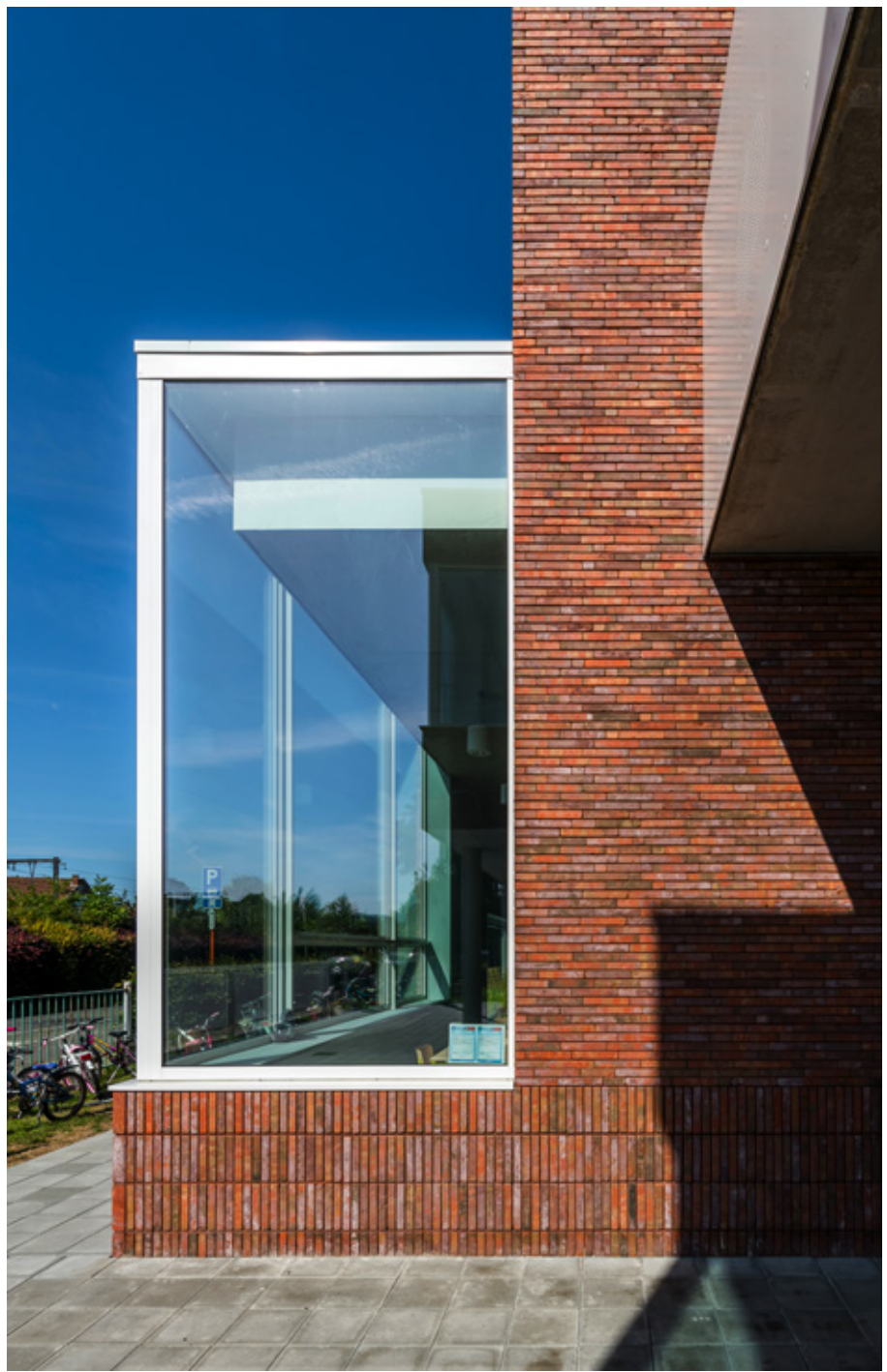
Metropolis Aula Red
