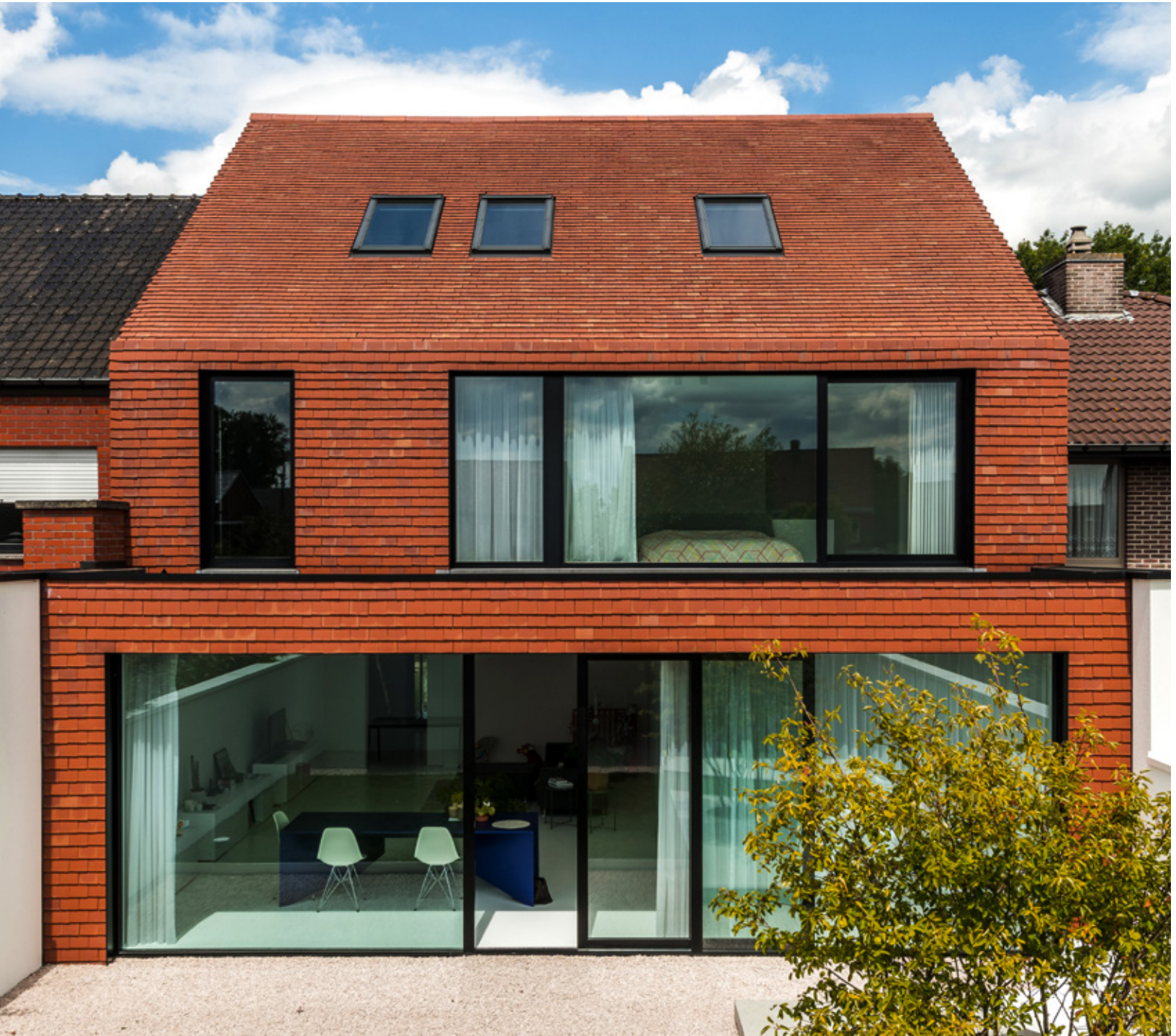
Façade and roof: Koramic Plain Tile Aléonard Pontigny Red Flamed
