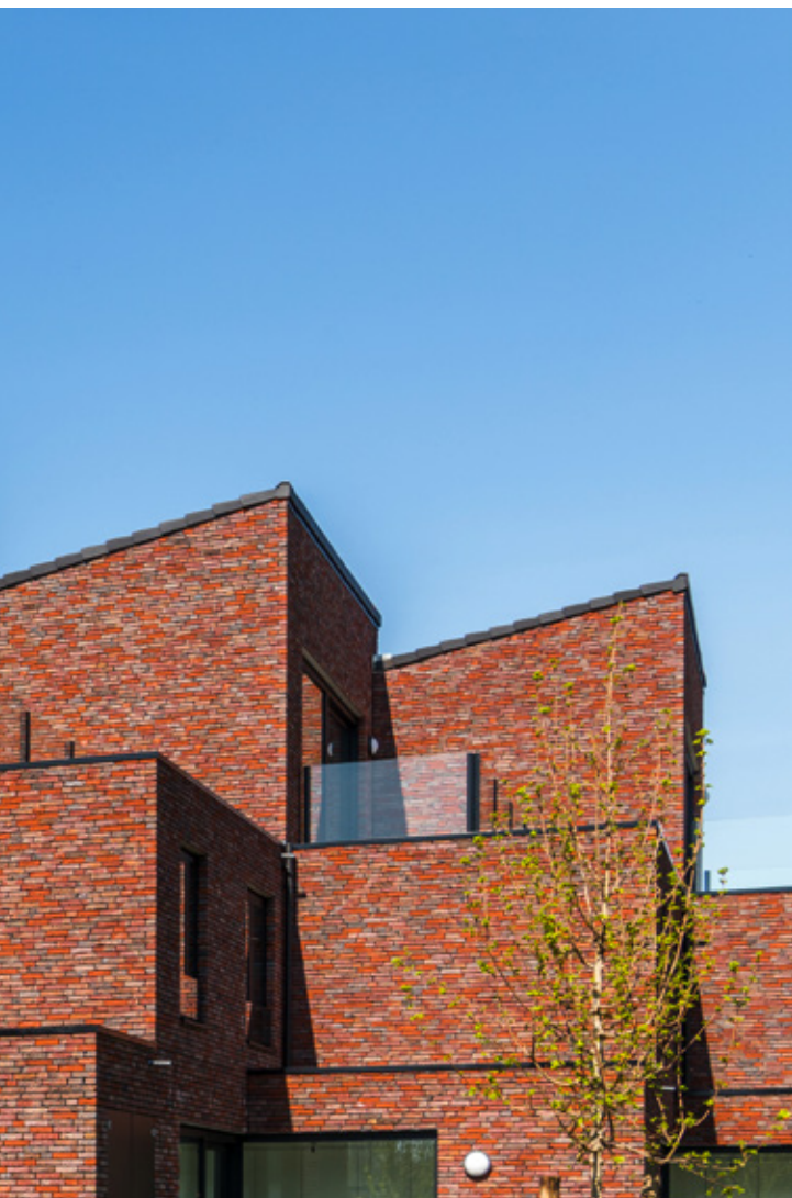
Façade: Brick mix Maaseiker Bont and Purple Blue Roof: Actua 10 Slate Engobe
