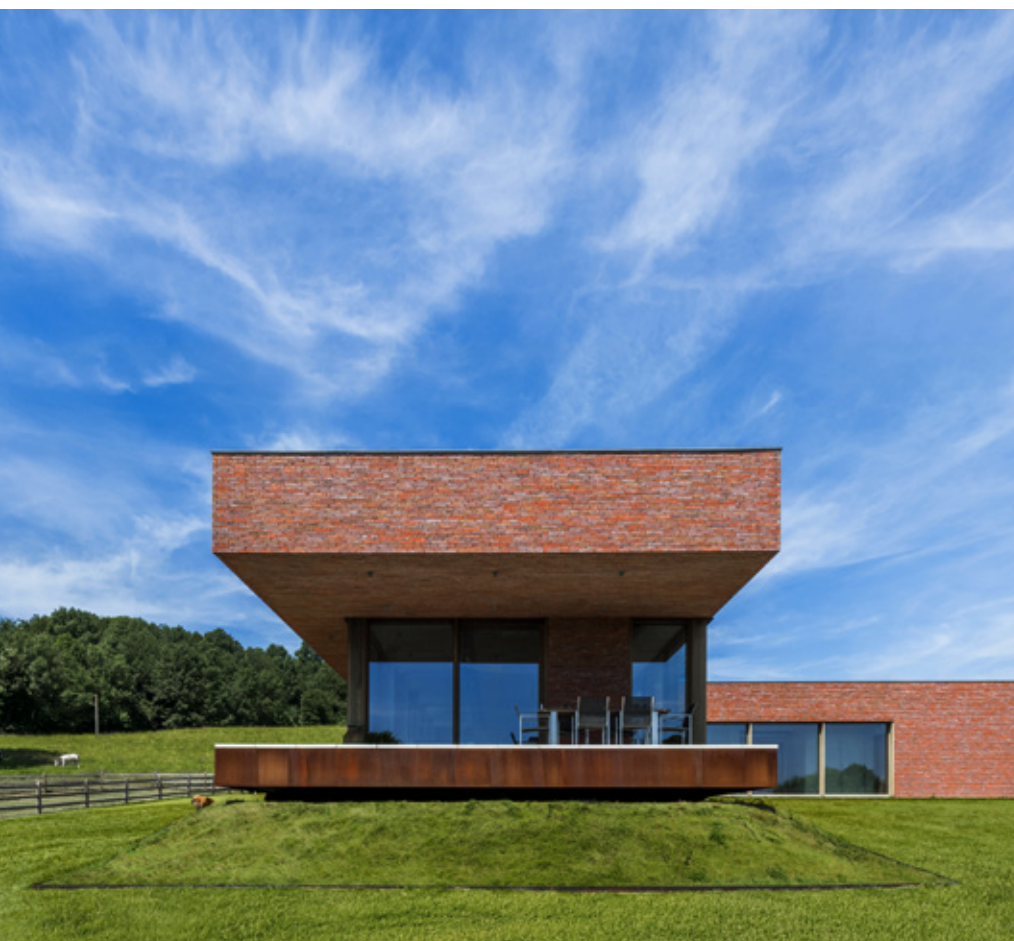
Metropolis Aula Red
