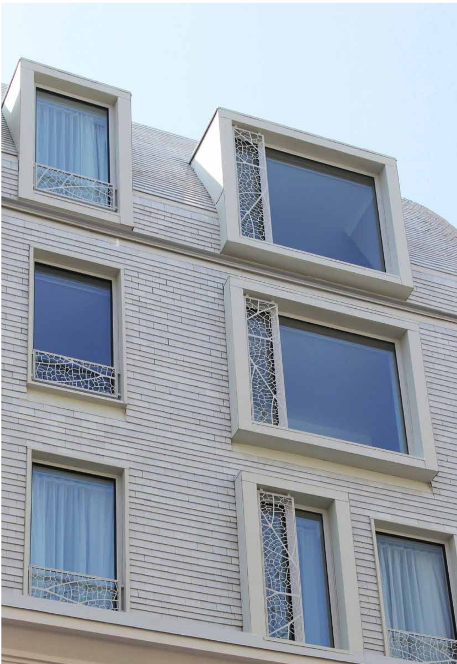
Koramic Plain Tile 301 White Glazed (roof and façade) Pierre Monmarson Architecture, FR-Paris
