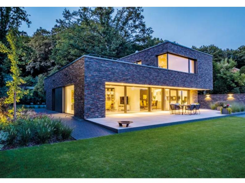
Space is gained with the narrow bricks. Furthermore, a narrower brick means less energy during firing, less clay, and lower resource costs.
